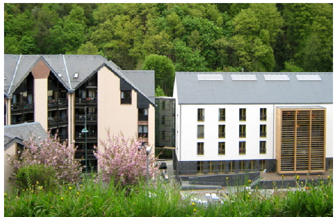
Ardennes Residence in Clervaux, Luxembourg (ARCHITECTURE ET ENVIRONNEMENT S.A.)
